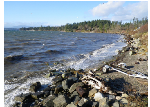
Patricia Bay - Example of degraded beach and rip rap.
